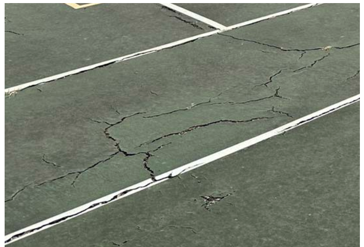
01_Weathered + Cracked Playing Surface
